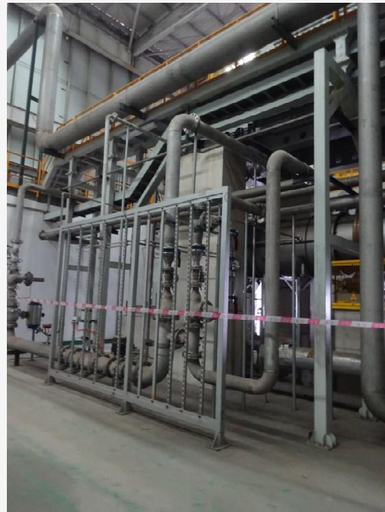
DRA 16/100-E-85 with separate Air Cooling Pipe CP12/120-A, increased O2-Atmosphere
